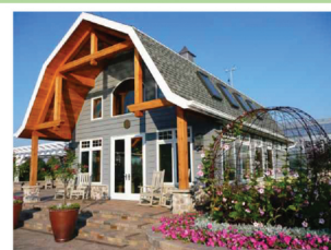
(Restrooms Inside) Greenhouse & Conservatory
